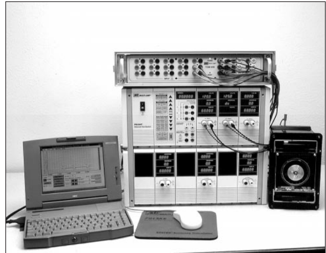
Figure 1: Testing Mechanical Reclosing Relay
